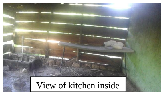
View of kitchen
