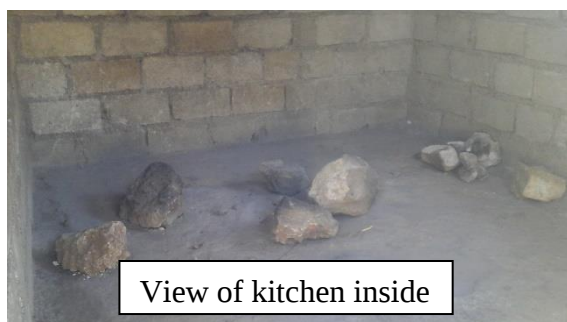
View of kitchen
