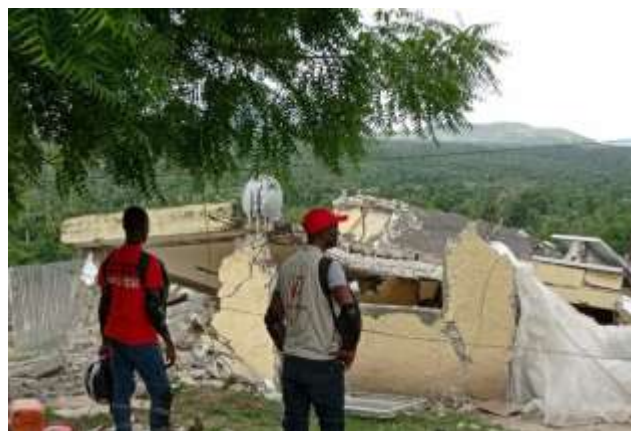
Rapid needs and damage assessment (Commune of l'asile, August 16, 2021)
