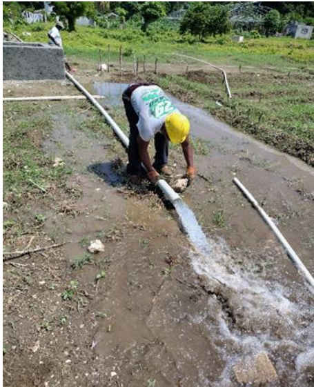
Installation of the new irrigation system at the ATP at FAMV.
