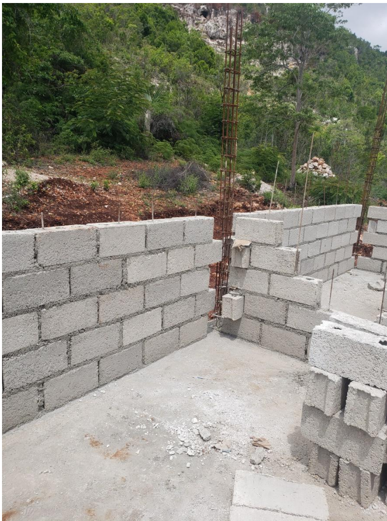
Figure 13. Masonry wall block elevation observed in progress- building 6.
