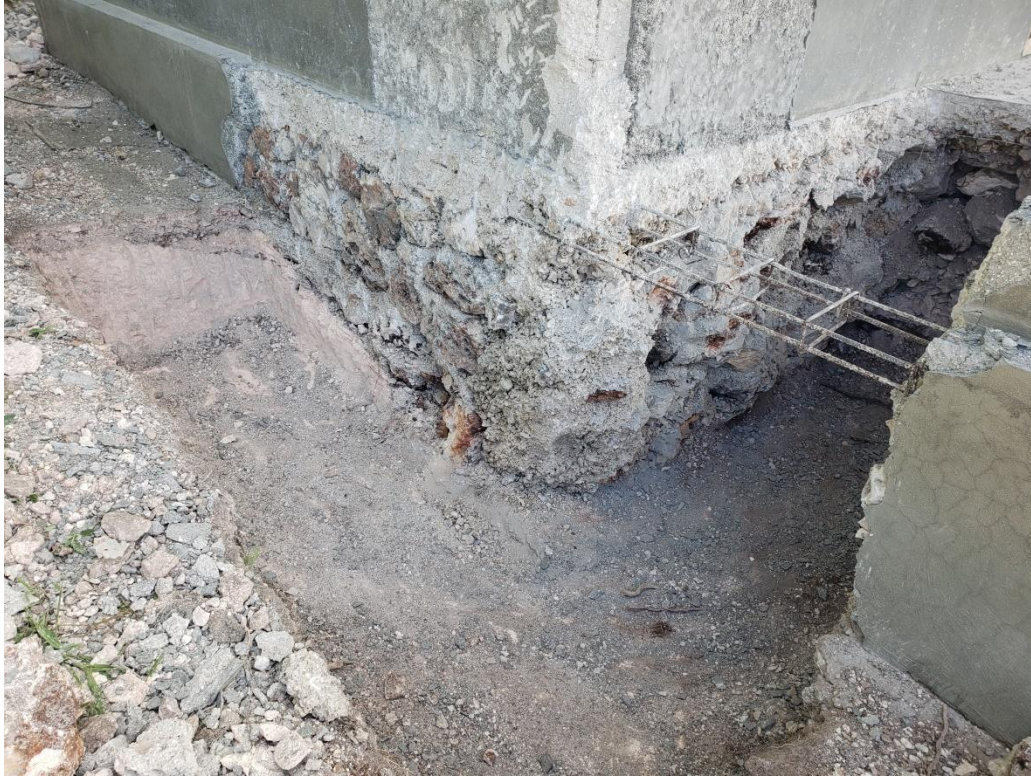
Figure 10. Footing excavation observed in progress- Building 6.
