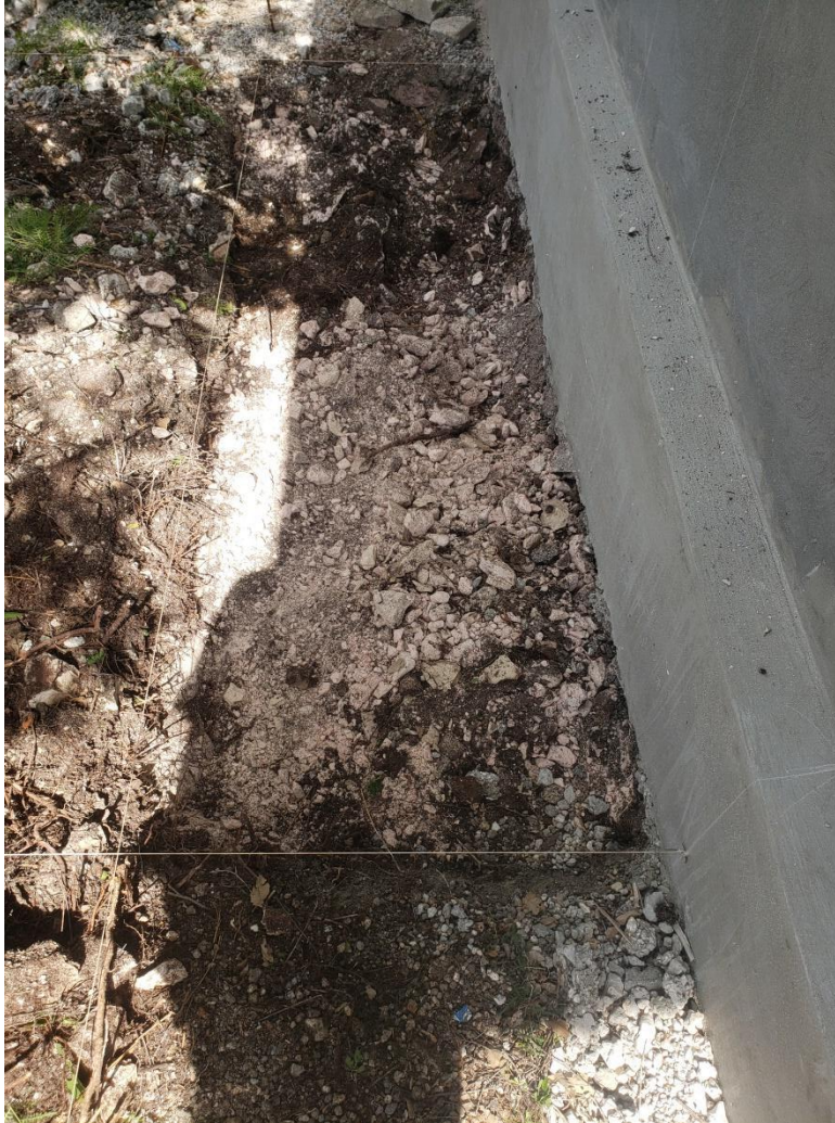
Figure 9. Footing excavation observed in progress-Buidling 5.
