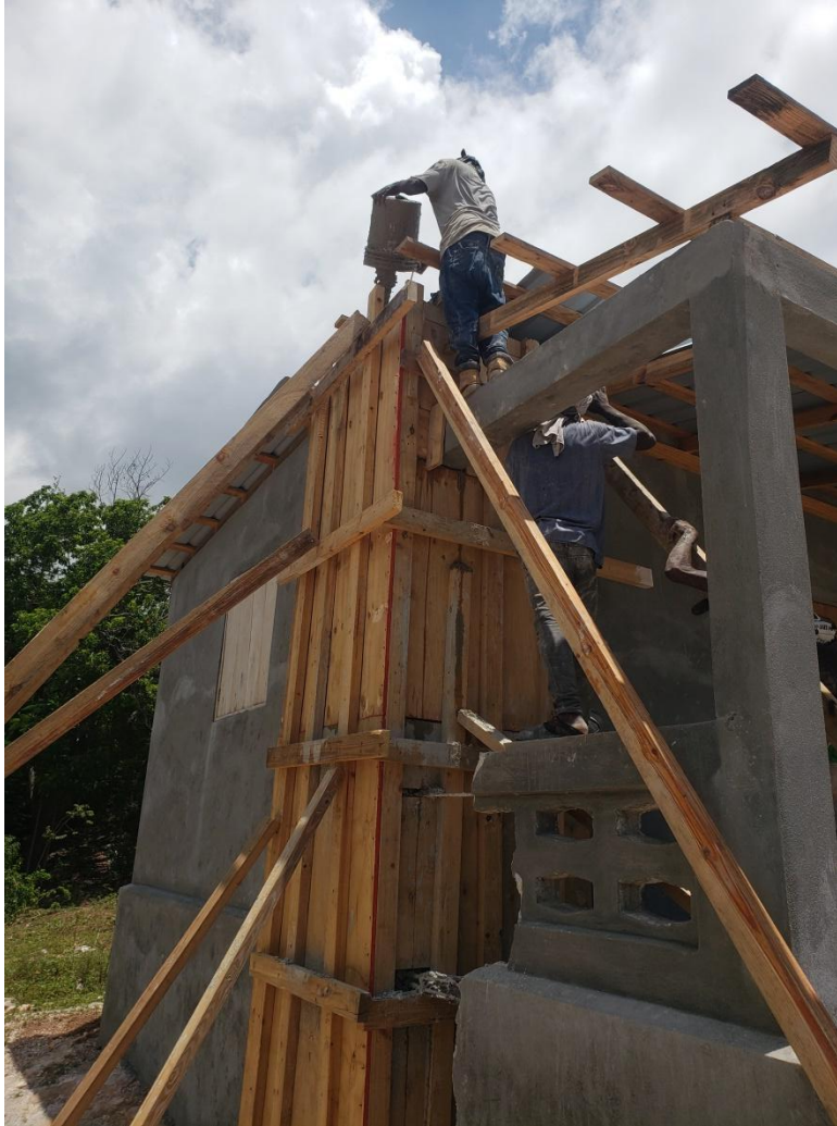
Figure 5. Shear wall concrete placement- Building I.
