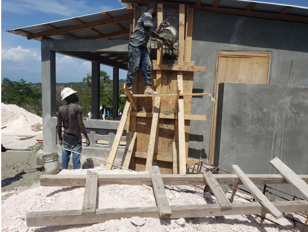
Figure 8. Shear wall concrete placement observed in progress.
