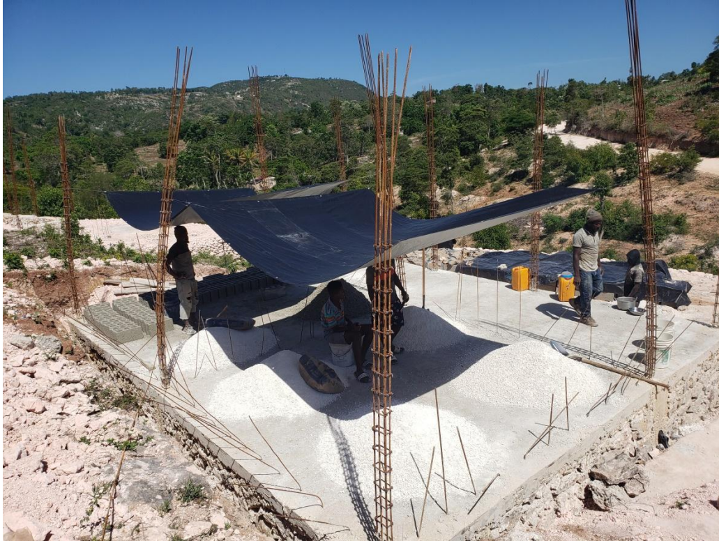
Figure 12. Storage of materials for concrete blocks production.
