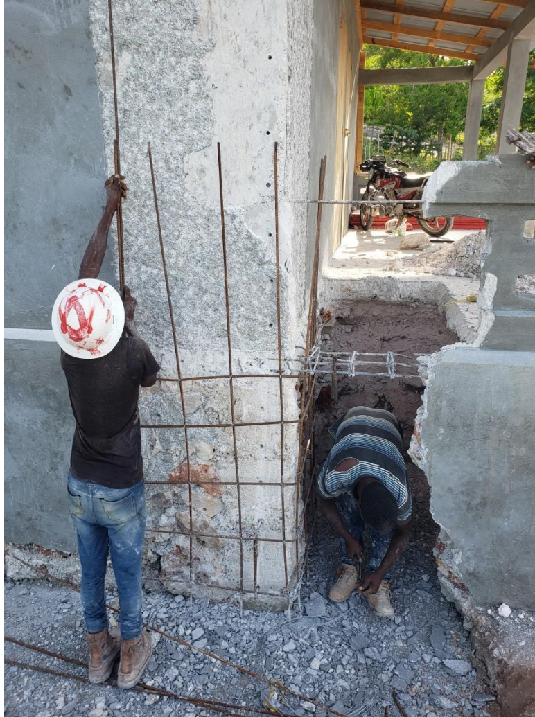
Figure 5. Shear wall reinforcing steel observed in progress.
