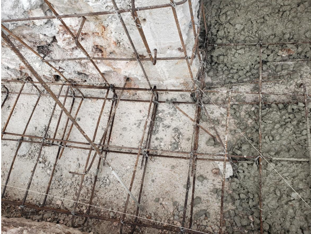
Figure 3. Example of foundation reinforcement and concrete placement.
