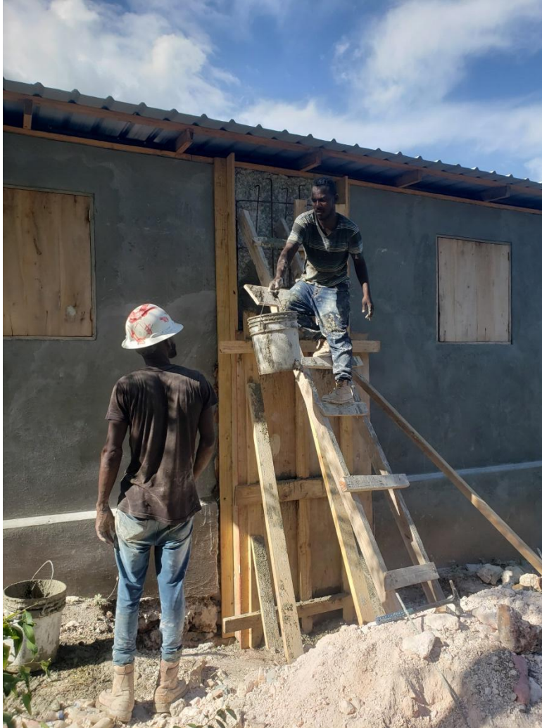
Figure 7. Example of shear wall concrete placement observed in progress.
