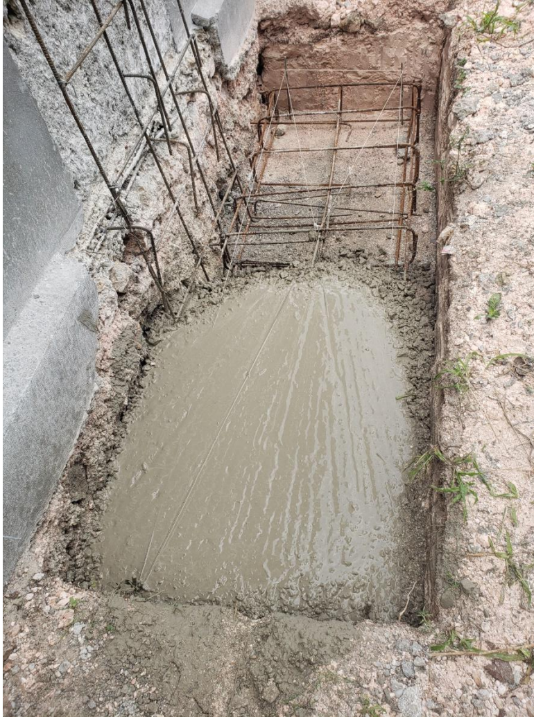
Figure 2. Example of foundation concrete placement observed.
