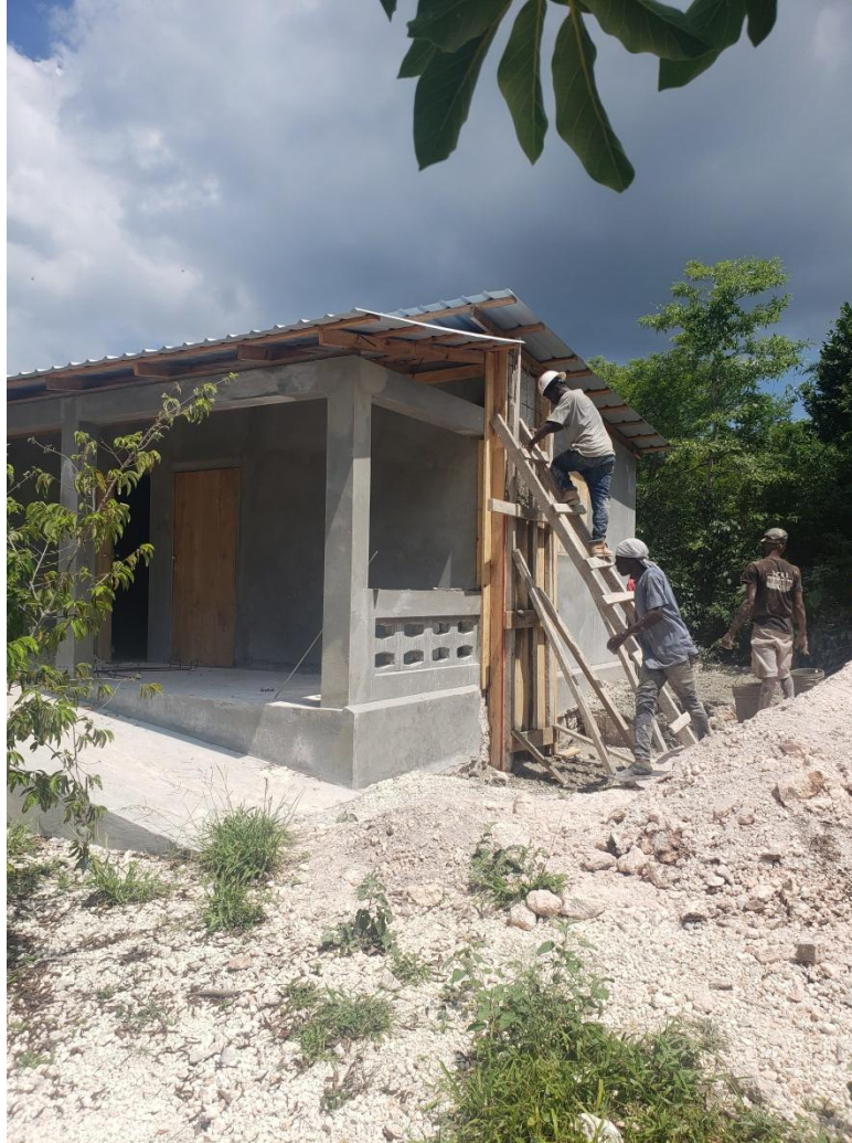
Figure 6. Shear wall concrete placement observed in progress- Buidling 2.
