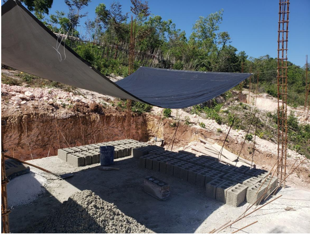
Figure 10. Production of concrete blocks.
