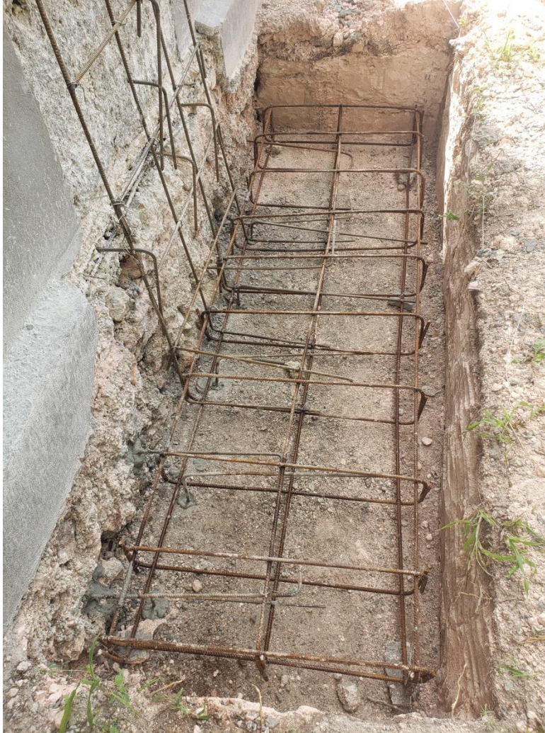
Figure 1. Example of foundation reinforcement in progress.
