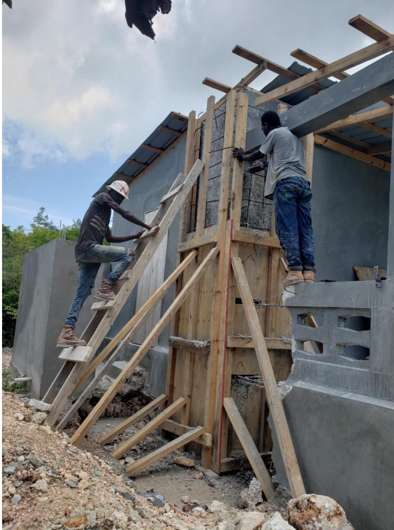
Figure 3. Example of shear wall reinforcement in progress.
