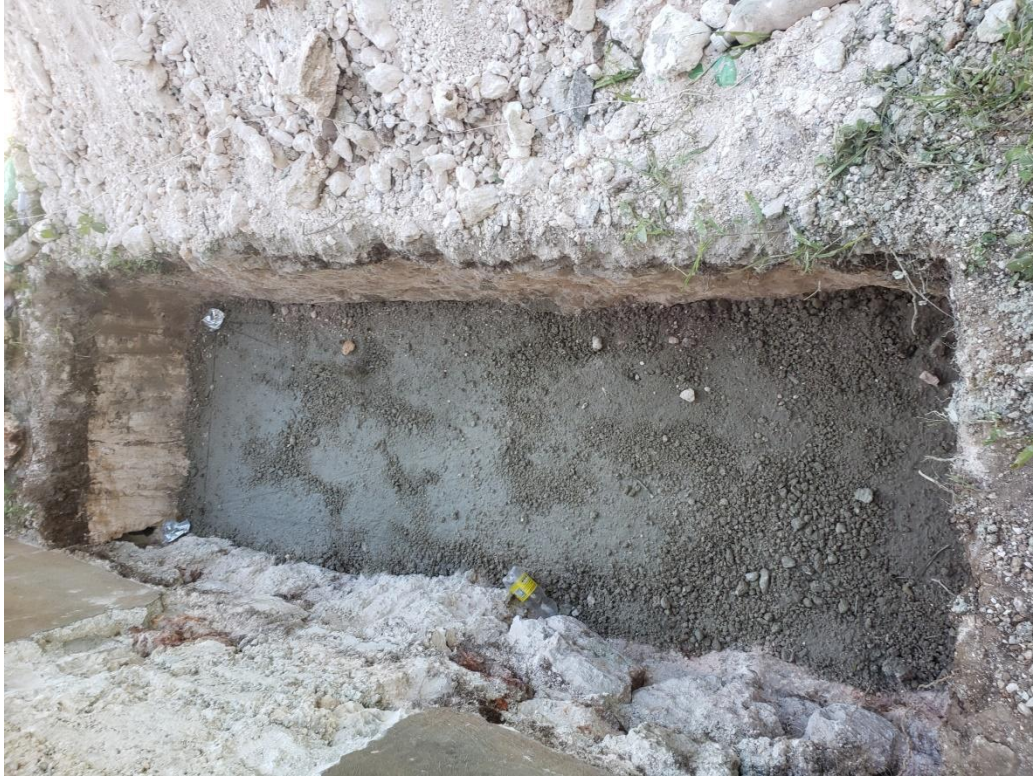
Figure 1. Foundation excavation and lean mix concrete placement.
