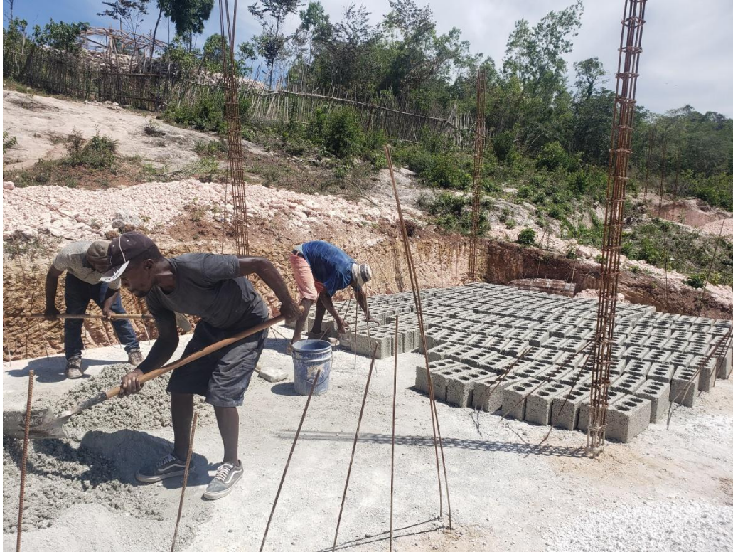
Figure 11. Production of concrete blocks.
