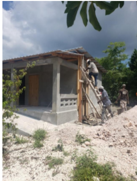
Construction on a house on La Gonâve
