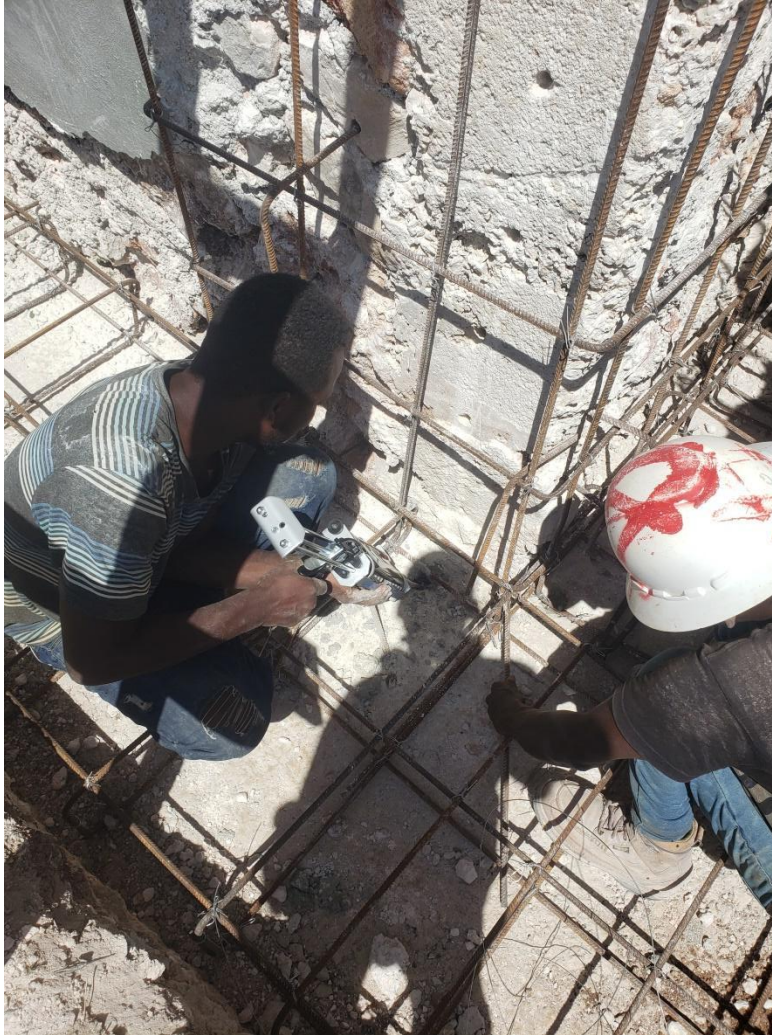
Figure 2. Example of foundation reinforcement in progress.
