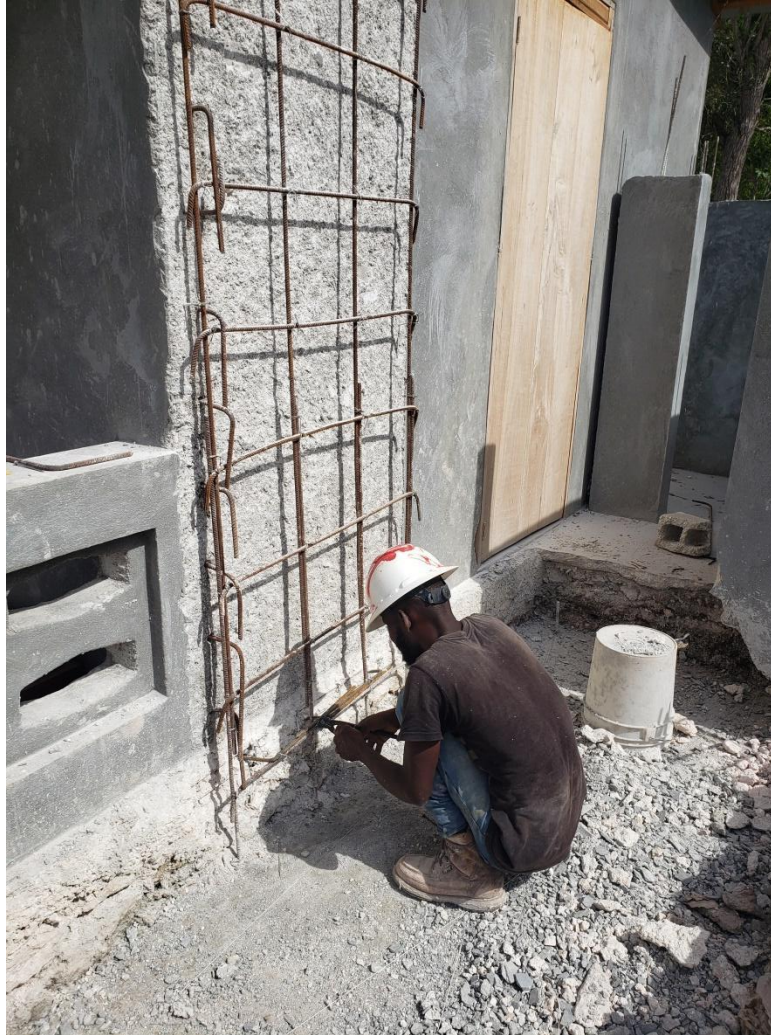
Figure 6. Cleaning the rebar before setting up the formwork.
