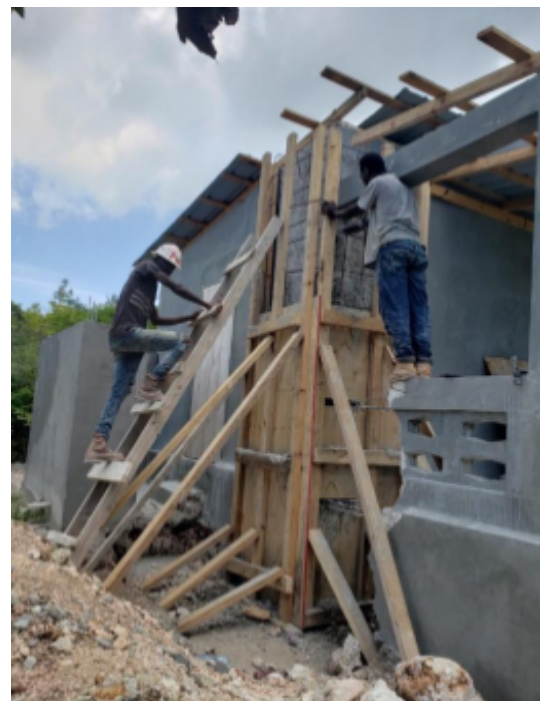
Construction on a house on La Gonâve
