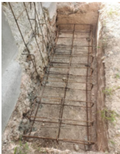
Shear wall foundation reinforcement in progress for a house in La Gonâve
