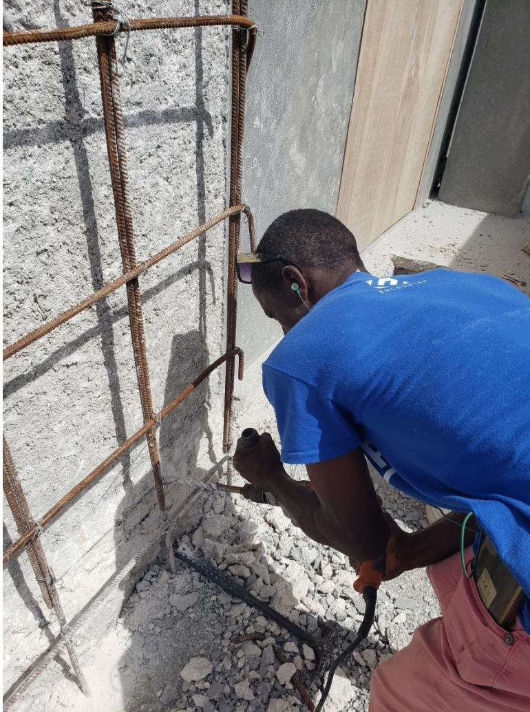
Figure 4. Drilling of the existing bond beam for epoxy dowel placement.
