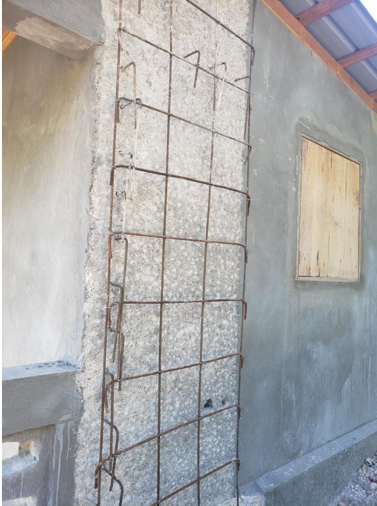
Figure 4. Example of shear wall reinforcement in progress.
