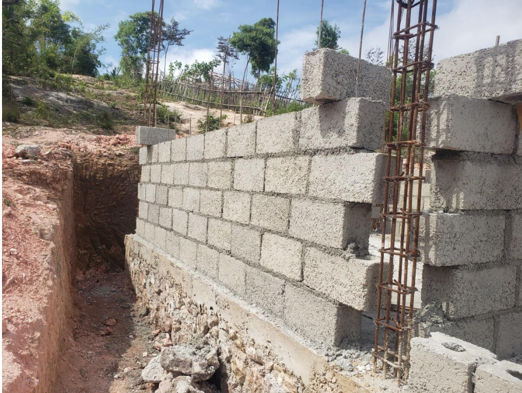
Figure 11. Masonry block wall elevation observed in progress- building 5.
