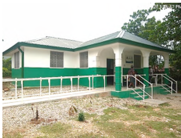
LABICHE MEDICAL CLINIC WAS FULLY RENOVATED TO REPAIR DAMAGE FROM HURRICANE MATTHEW
