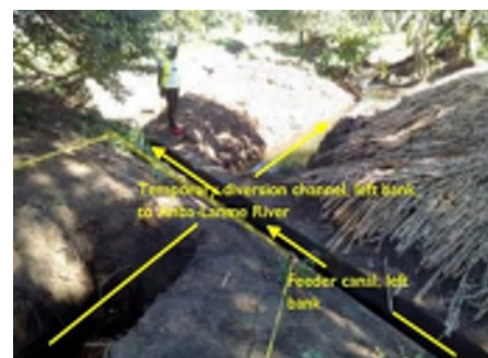
AECOM PROVIDED ANNOTATED VISUALS TO AID COMMUNICATION OF ISSUES AND WORK PROGRESS
