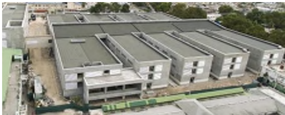
HUEH POST-AECOM SERVICES, NEARING COMPLETION
