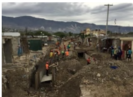
AECOM PROVIDED QUALITY ASSURANCE INSPECTIONS THROUGHOUT CONSTRUCTION
