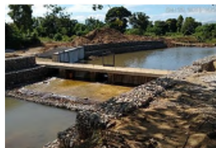
THE CHALOPIN SYSTEM REHABILITATION WAS COMPLETED IN 2020, PROVIDING FARMERS WITH INCREASED ACCESS TO IRRIGATED LAND
