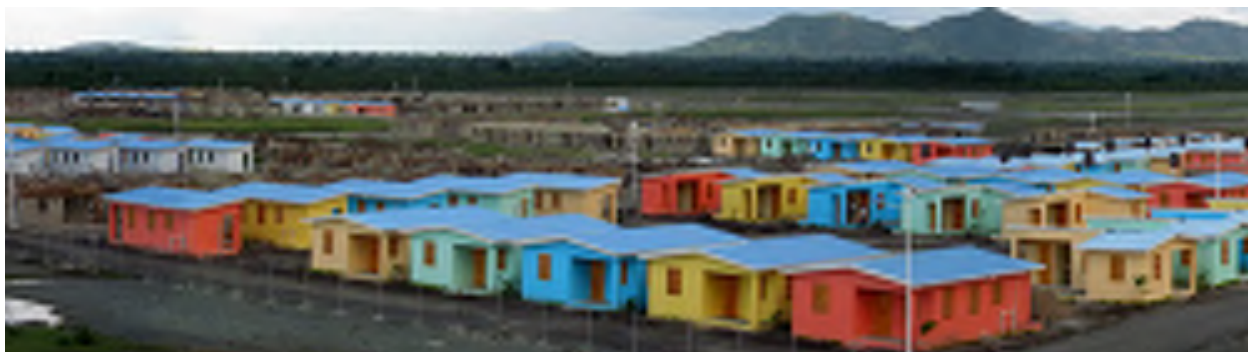
SUPPORTING USAID IN ASSESSING NEEDED REPAIRS TO THE SEPTIC SYSTEM AT THE EKAM DEVELOPMENT IN CARACOL
