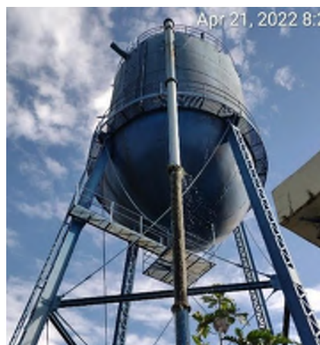
WATSAN INCLUDED A WIDE RANGE OF PROJECTS: TOP: INSPECTING A WATER KIOSK UNDER CONSTRUCTION MIDDLE: INSTALLATION OF NEW HDPE TRANSMISSION PIPES IN LES CAYES BOTTOM: LEAK INSPECTION AT THE CHARPENTIER WATER TANK
