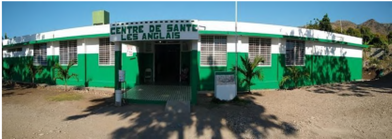
AECOM PROVIDED EARTHQUAKE DAMAGE ASSESSMENT AT LES ANGLAIS MEDICAL CLINIC AND HELPED USAID DEVELOP CONTRACT CHANGES TO INCLUDE THESE REPAIRS IN THE CONTRACTOR'S SCOPE
