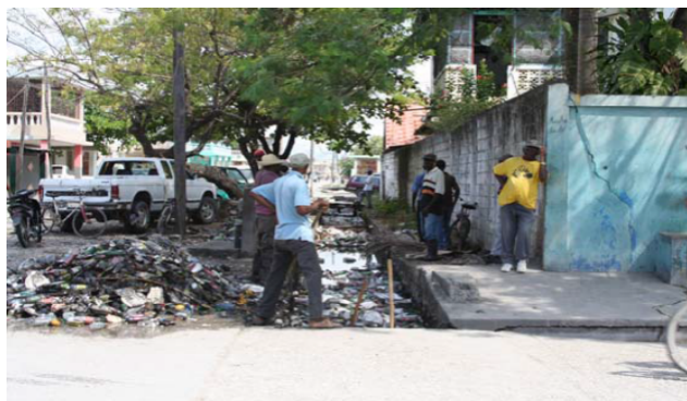
FIGURE 5: NETTOYAGE DRAINAGE EXISTANT
