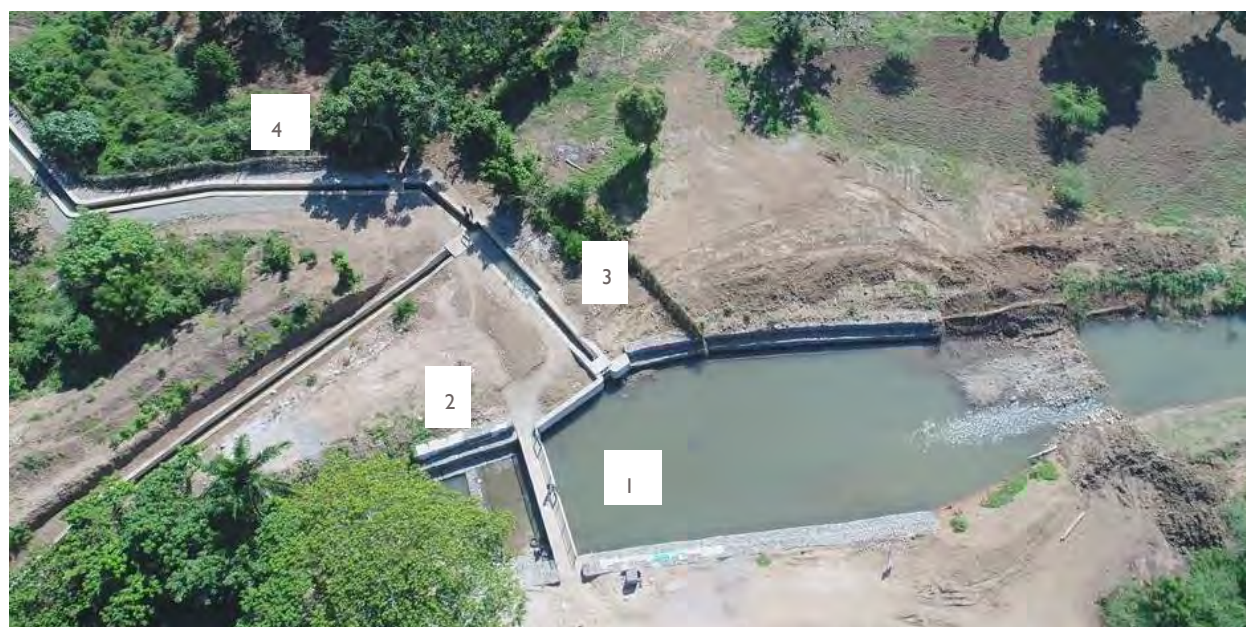
Figure 5: Chalopin Irrigation System seen from above (1. diversion structure, 2. escape canal, 3. sedimentation basin, 4. primary canal) Photo Credit: Eric Auguste for MARNDR
