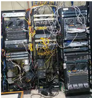
Before its renovation, the NOC's server boxes and cords lacked organization.
