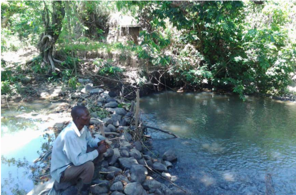
FIGURE 23: JANM PANTALON DIVERSION ON THE MARION RIVER WITH MARION ON THE LEFT AND THE CHANNEL TO MALFETY-CHALOPIN ON THE RIGHT (SOURCE: SOCIÉTÉ D'EXPERTISE ET D'INGÉNIERIE LGL SA, 2013)
