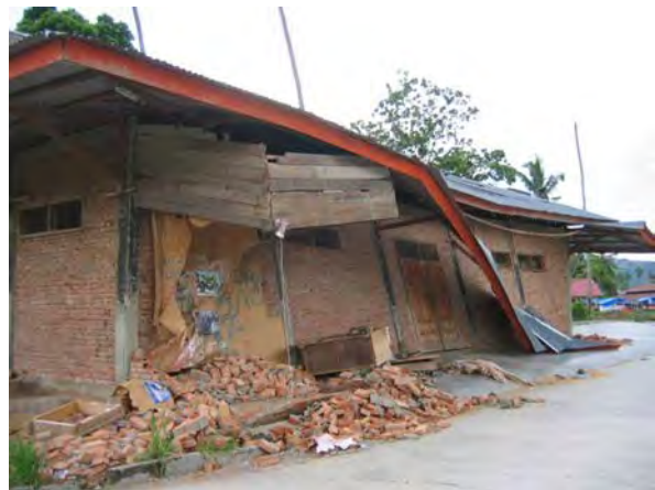
Figure 12. Confined masonry warehouse with out-of-plane failure of long walls without cross-bracing, , IMG 8891
