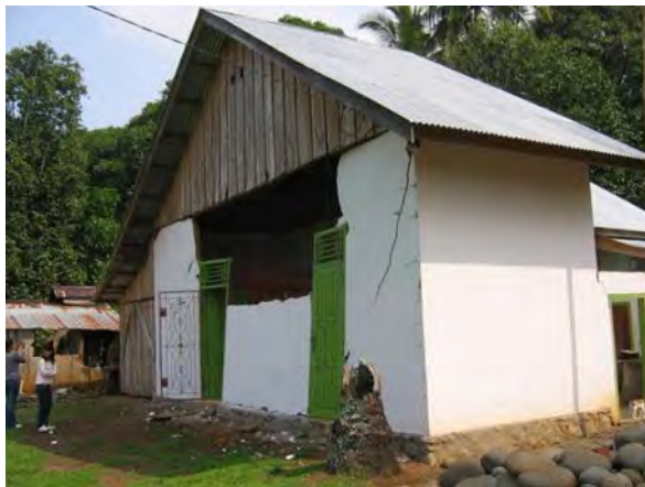
Figure 11. Confined masonry building with overturning failure of tall, unsupported wall, Kec. Airnapal (North Bengkulu)
