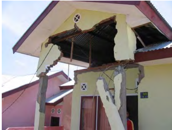
Figure 13. Subdivision of confined masonry houses, damage to covered terrace, Bengkulu. S3.83218° E102.29287
