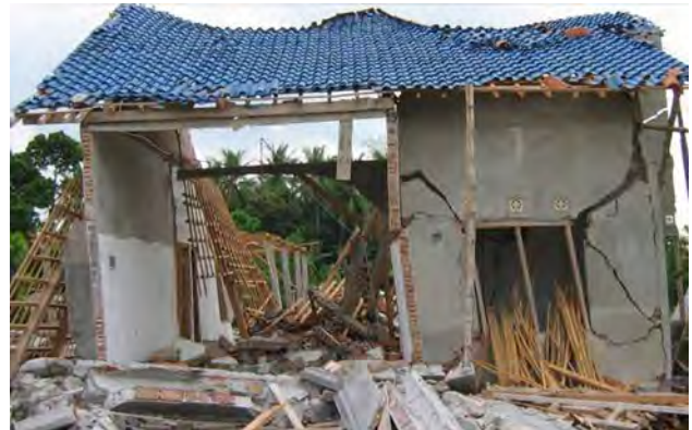
Fig. 3. Confined masonry house under construction, insufficient connections, Pleret (Bantul). S7.87574°, E110.40703°, IMG_6575
