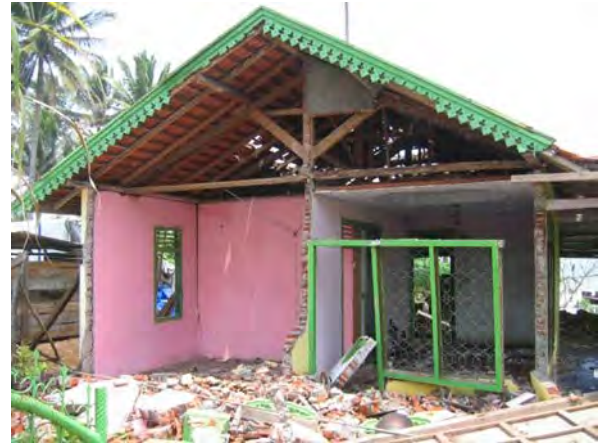
Figure 9. Partially collapsed brick masonry house with reinforced concrete (RC) tie columns and timber bond beams, note partial collapse of masonry gable wall, and lack of in-plane stiffness in front wall, Kec. Lais (North Bengkulu) S3.53217° E102.03771
