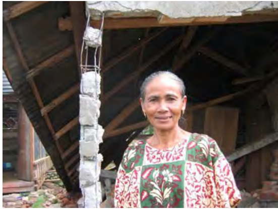
Figure 24. Homeowner standing in front of her collapsed wall, note quality of concrete, Padang Panjang, IMG_8840.
