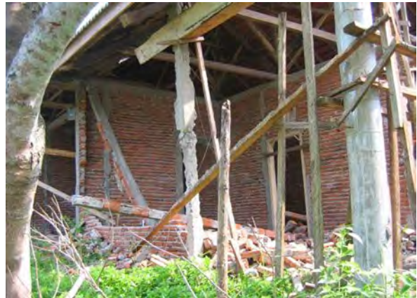
Figure 22. Confined masonry house with failure in masonry walls and connections between tie columns and bond beams, Kec. Airnapal (North Bengkulu)
