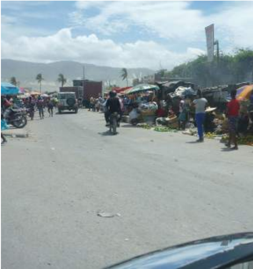
Fig.10: Existing national road in Canaan.
