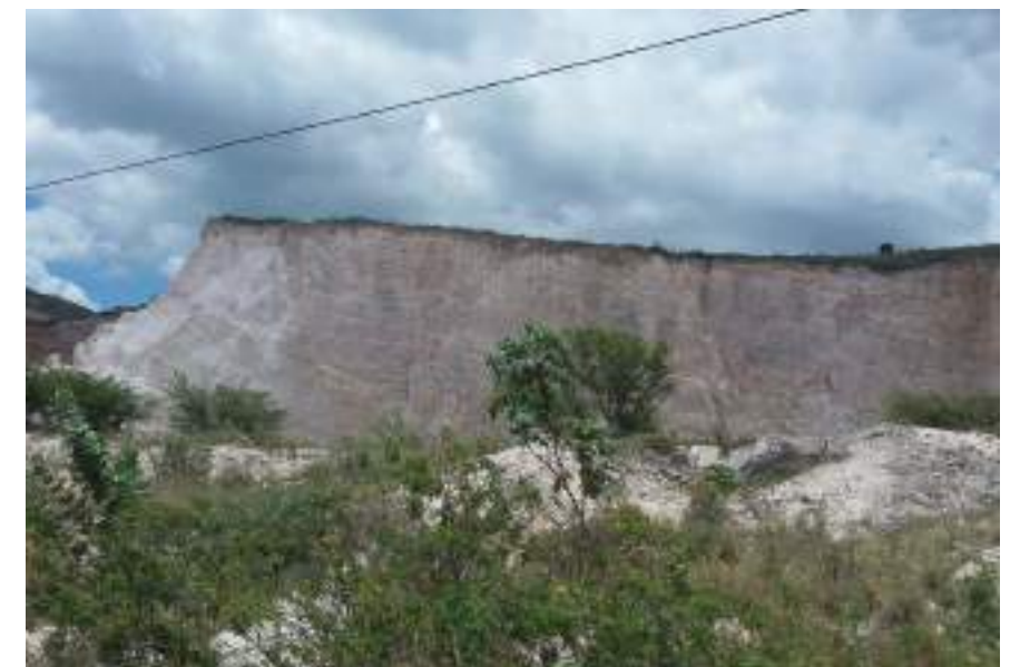
Fig.34: Abandoned quarry in Canaan
