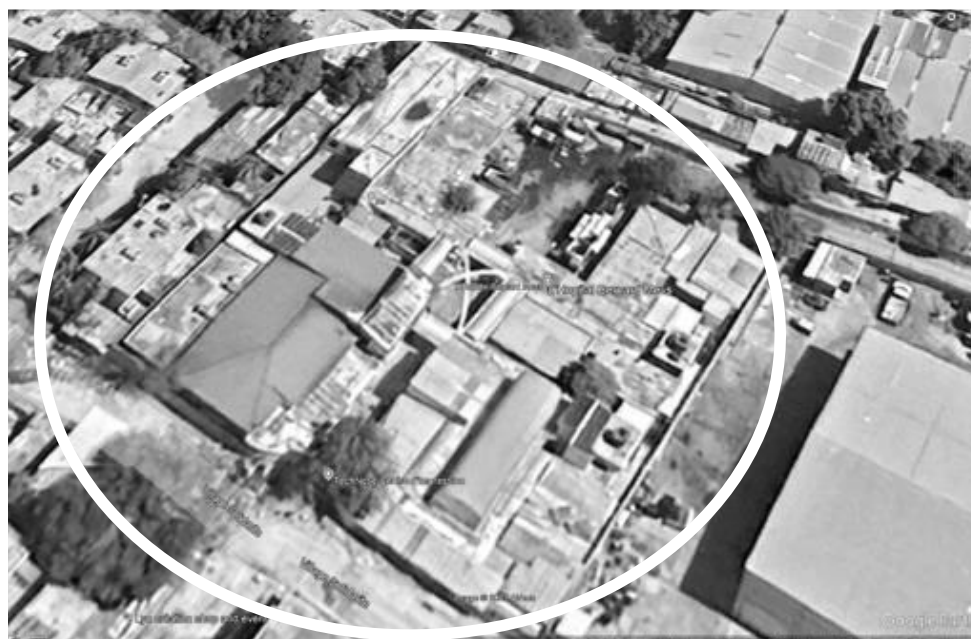
Figure 2. Bernard Mevs Hospital satellite image taken 15 March 2025.
