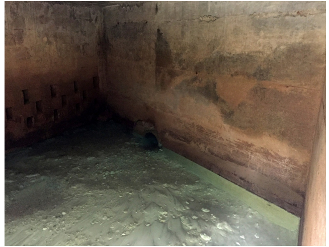
Photo 8. East outlet to pumping station.
