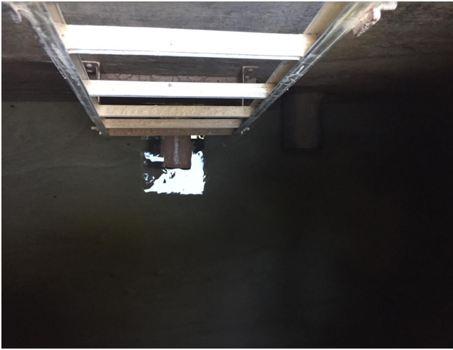
Photo 7. West outlet to pumping station.
