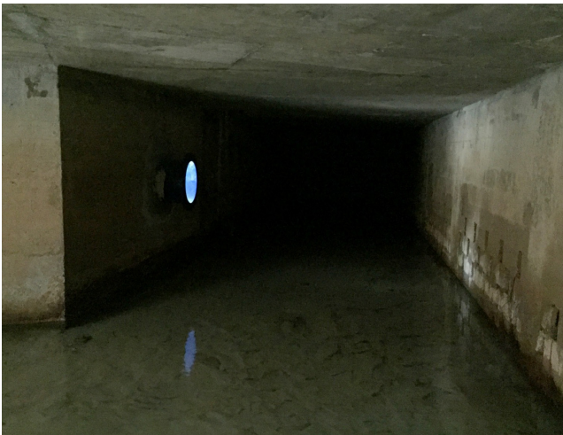
Photo 9. Inside view, overflow portal to surface drainage.
