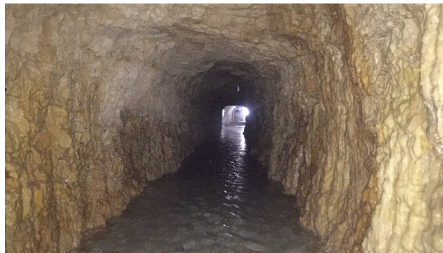
Photo 1. Limestone exposed in the main tunnel.
