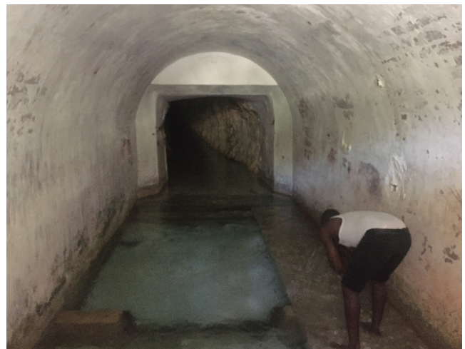
Photo 1. View inside tunnel portal.
