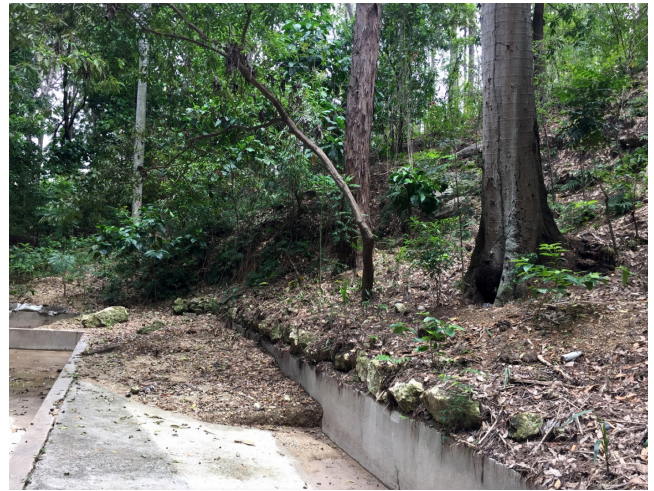
Photo 16. Clean-up in progress to remove fallen debris from slope above catchment.
