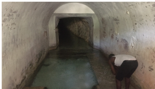
Photo 2. The tunnel portal facing into the tunnel.
