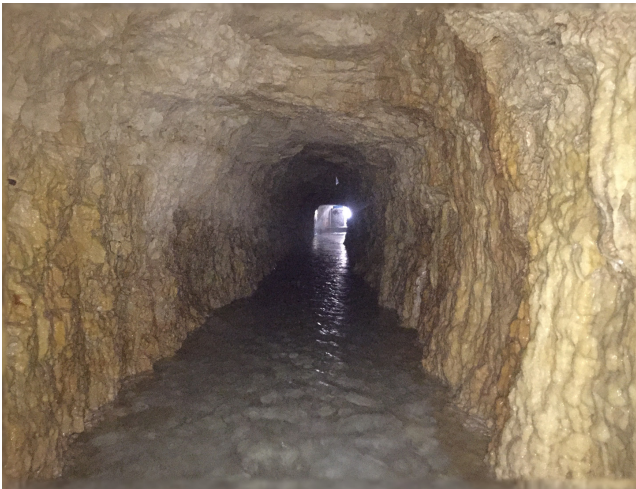
Photo 3. View of limestone geology looking toward tunnel portal.
