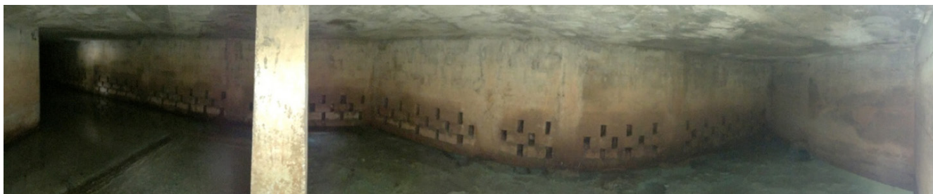
Photo 6. Panoramic view of inside spring catchment, outlet to distribution at bottom right.
