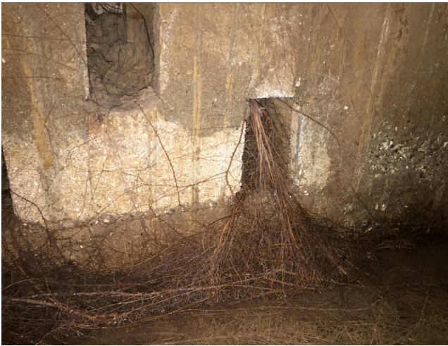
Photo 15. Roots entering the spring catchment.
