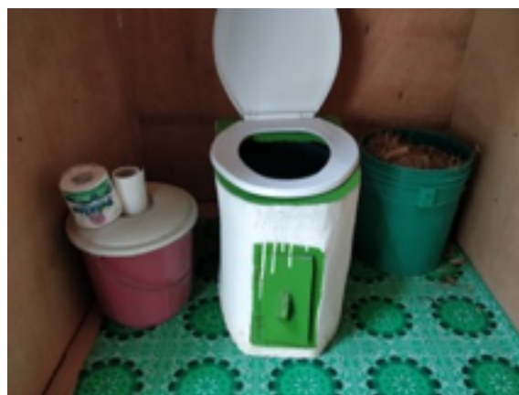
Figure 14. SOIL CBS toilet and cover material (sugarcane bagasse) on the right. Photo credit: SOIL
