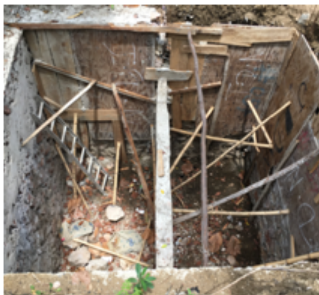
Figure 9. New construction of two-compartment pit for a health clinic, commonly referred to as septic tank in Cap-Haïtien. Photo credit: Anthony Kilbride
