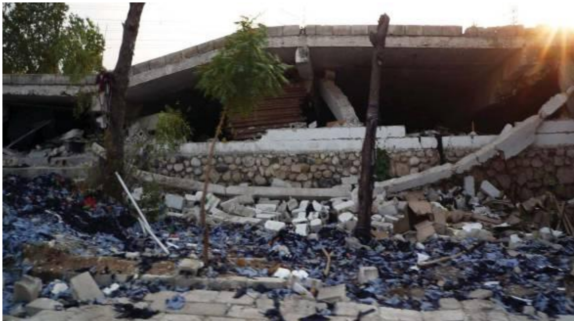
Photo 1: Collapsed building in Delmas, Port-au-Prince
