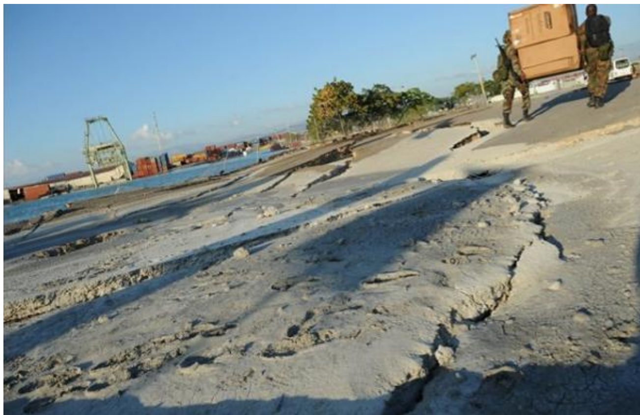
Photo 4. Liquefaction (sand extrusions and lateral spread) of sandy soils in the Port-au-Prince port area
