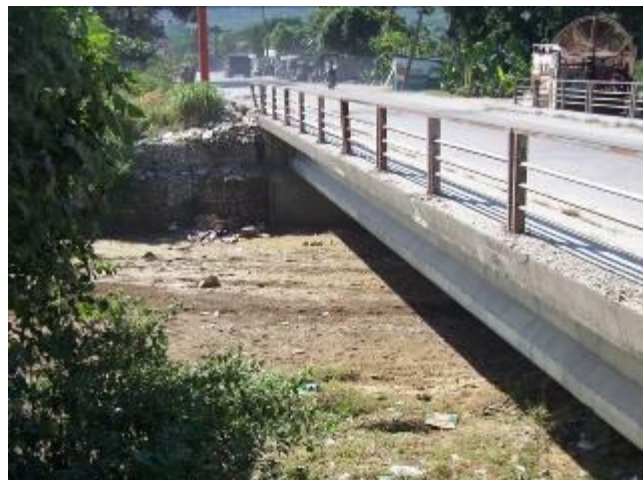
Photo 12. Rouyonne river, Léogane. Very limited water flow space under the bridge of the national highway owing to gravel build-up in the low-flow channel. Source: Predict Services, December 2009
