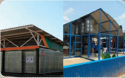
STATIONS D'EAU Water Kiosk STATIONS VERTES Green Stations
