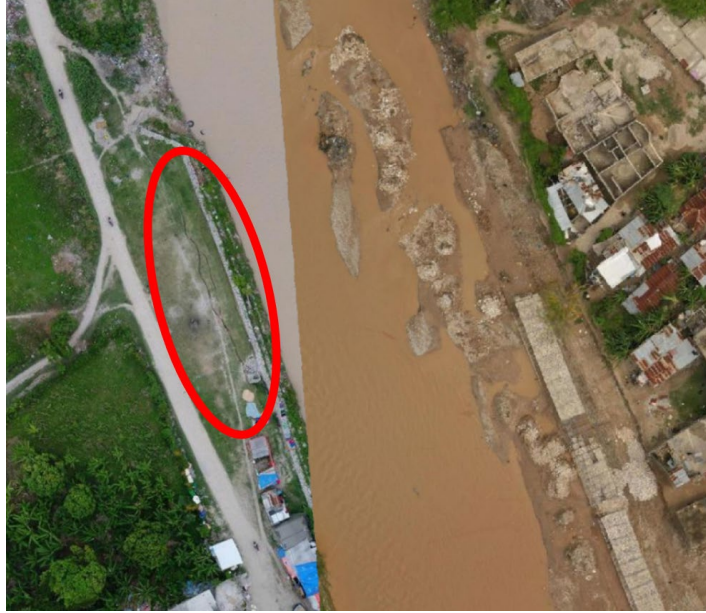
Figure 7.93. Damage and possible lateral spreading near river (Ravine du Sud) in Les Cayes. Coordinates: 18.195 -73.760278. Images courtesy of OpenstreetMap (Pierre Béland, https://pierzen.dev.openstreetmap.org/ ).
