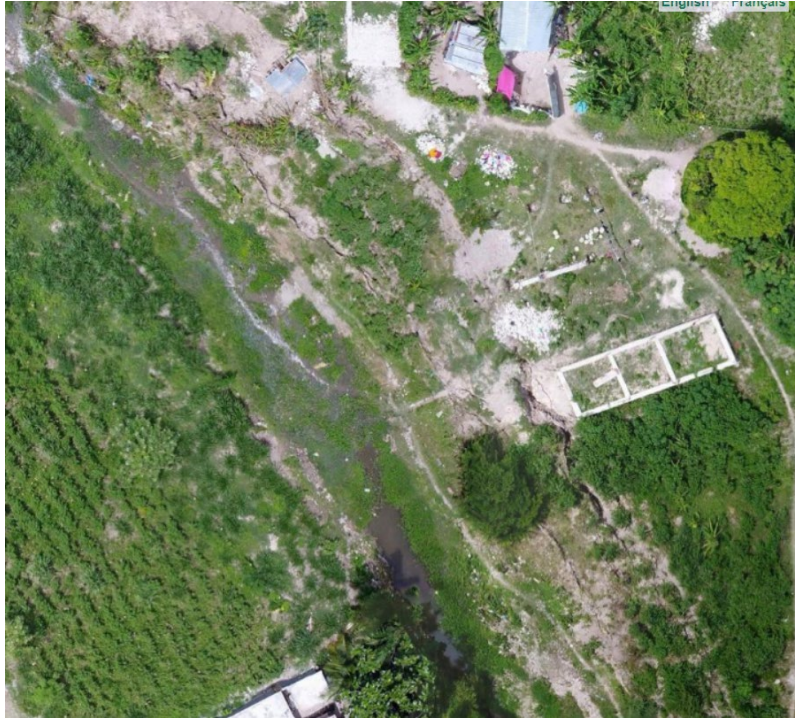
Figure 7.95. Damage and possible lateral spreading near river (Madan Samdi) in Les Cayes. Coordinates: 18.218333, -73.759444. Images courtesy of OpenstreetMap (Pierre Béland, https://pierzen.dev.openstreetmap.org/ ).
