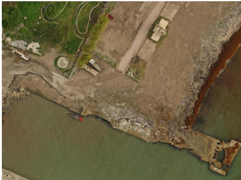
Figure 7.88. Coastal damage and possible evidence of liquefaction-induced lateral spreading in south Les Cayes. Coordinates: 18.189722, -73.748333. Images courtesy of OpenstreetMap (Pierre Béland, https://pierzen.dev.openstreetmap.org/ ).
