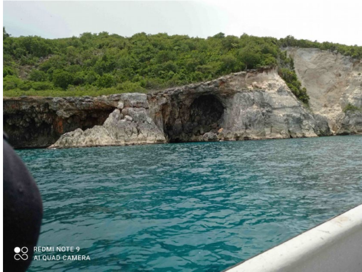
Figure 7.77. Rockfall along northern coast of southern peninsula of Haiti (Lat: 18.5925, Lon: - 73.95222). Photo taken September 29, 2021, courtesy of Dr. Newdeskarl Saint Fleur.
