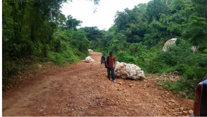
Figure 7.66. Rockfall along Highway 218 near Pestel (Lat: 18.5323424, Lon: -73.7988606)
