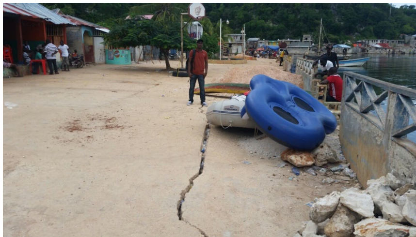
Figure 7.84. Ground cracking near the coast in Pestel (Lat: 18.5423509, Lon: -73.7906552).
