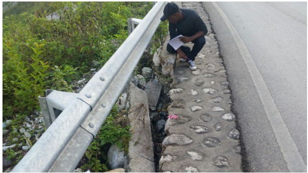
Figure 7.108. Pavement damage on RN7 (Lat: 18.4073805, Lon: -73.8794886).
