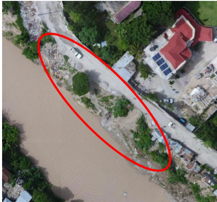
Figure 7.94. Damage and possible lateral spreading near river (Ravine du Sud) in Les Cayes. Coordinates: 18.196389, -73.760833. Images courtesy of OpenstreetMap (Pierre Béland, https://pierzen.dev.openstreetmap.org/ ).
