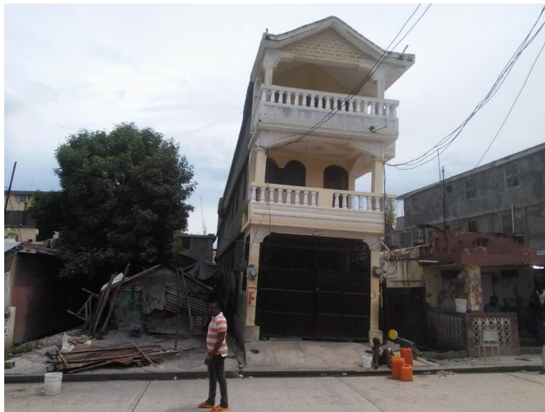
Figure 7.112. Damaged building in Les Cayes (Lat: 18.1956, Lon: -73.7456).
