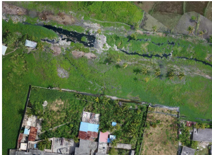
Figure 7.90. Possible lateral spreading in Les Cayes. Coordinates: 18.198611, -73.745833. Images courtesy of OpenstreetMap (Pierre Béland, https://pierzen.dev.openstreetmap.org/ ).
