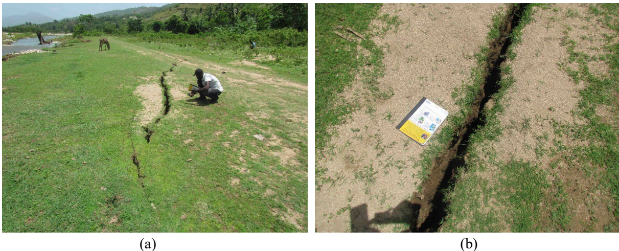
Figure 7.17. Surface cracks with evidence of sand ejecta immediately adjacent to the cracks (Lat: 18.35, Lon: -73.70694). Photos taken on August 28, 2021, courtesy of Dr. Newdeskarl Saint Fleur.
