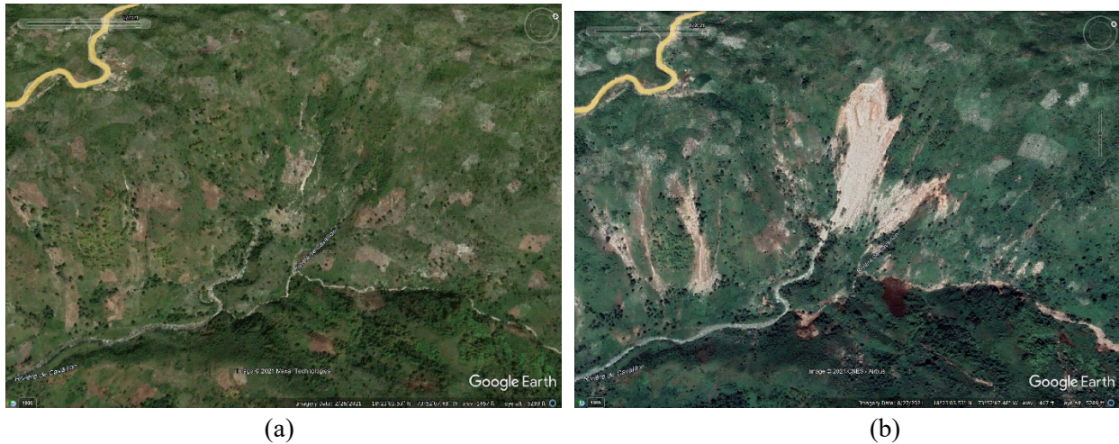
Figure 7.41. Landslide near RN7 with an average slope 47% over length of \sim 0.4 km as measured in Google Earth (18.385256, Lon: -73.869594). (a) February 26, 2021. (b) August 27, 2021.
