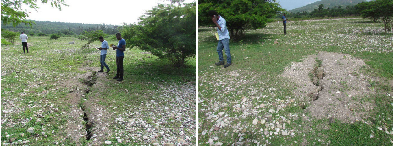
Figure 7.16. Surface cracks with evidence of sand ejecta immediately adjacent to the cracks (Lat: 18.38574, Lon: -73.41023). Photos taken on August 25, 2021, courtesy of Dr. Newdeskarl Saint Fleur.
