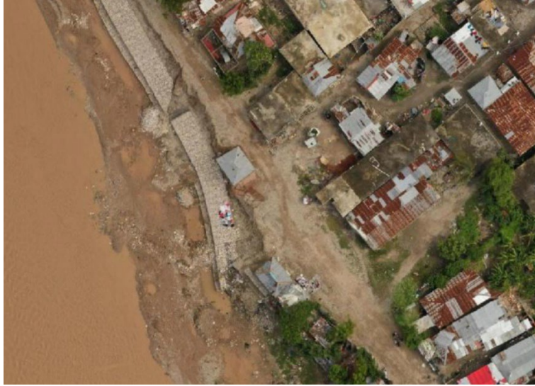
Figure 7.91. Damage and possible evidence of liquefaction-induced lateral spreading near river (Ravine du Sud) in Les Cayes. Coordinates: 18.195556, -73.759722. Images courtesy of OpenstreetMap (Pierre Béland, https://pierzen.dev.openstreetmap.org/ ).
