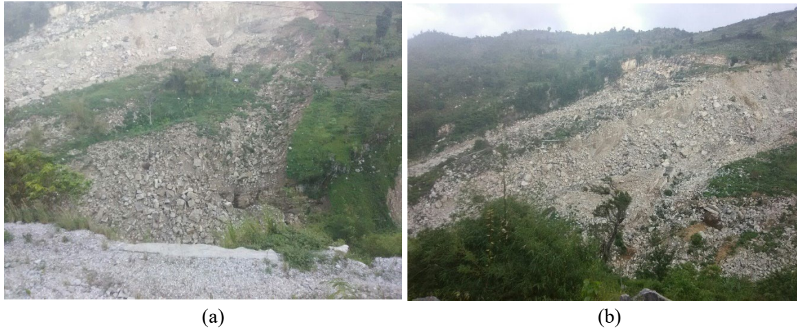
Figure 7.59. Possible landslide with boulder debris that may have occurred sometime prior to the August 14 earthquake, judging based on satellite imagery (Lat: 18.429649, Lon: -73.899932).
