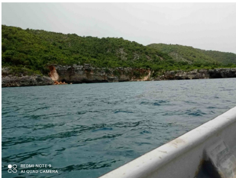
Figure 7.78. Rockfall along northern coast of southern peninsula of Haiti (Lat: 18.60111, Lon: - 73.96167). Photo taken September 29, 2021, courtesy of Dr. Newdeskarl Saint Fleur.
