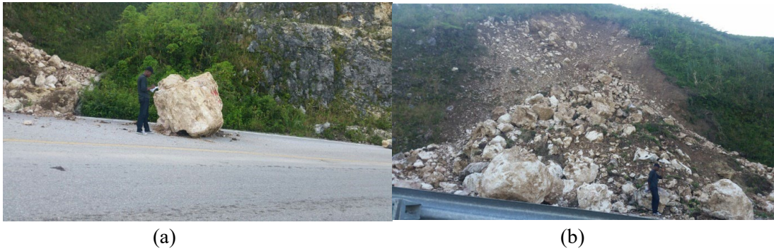
Figure 7.47. Landslide with boulder debris along RN7 (Lat: 18.4072403, Lon: -73.8819915).
