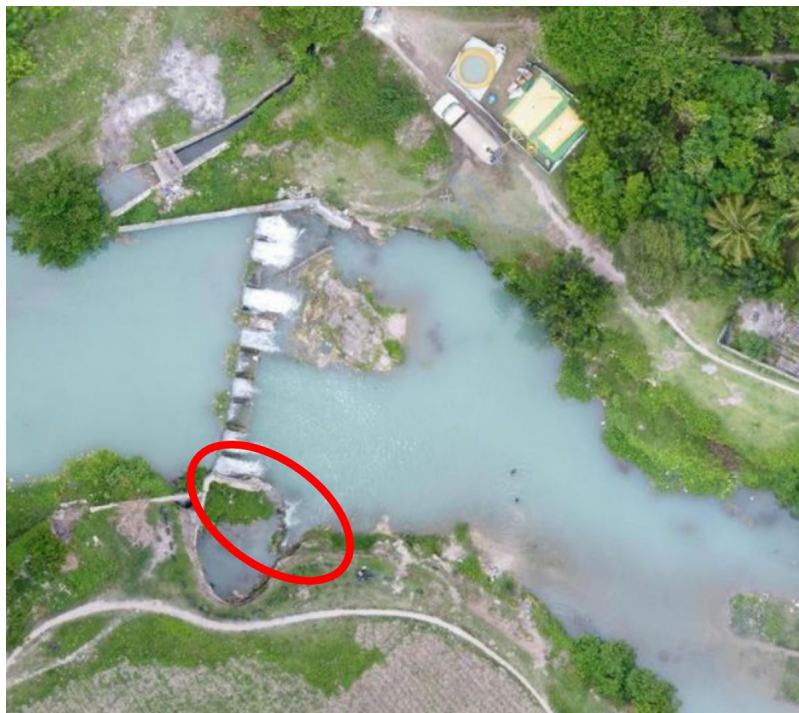
Figure 7.96. Possible damage of water facility near river (Riviere L'Islet) in Les Cayes. Coordinates: 18.215278, -73.745833. Images courtesy of OpenstreetMap (Pierre Béland, https://pierzen.dev.openstreetmap.org/ ).
