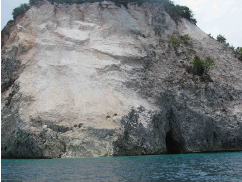
Figure 7.75. Rockfall along northern coast of southern peninsula of Haiti (Lat: 18.59556, Lon: - 73.94944). Photo taken September 29, 2021, courtesy of Dr. Newdeskarl Saint Fleur.
