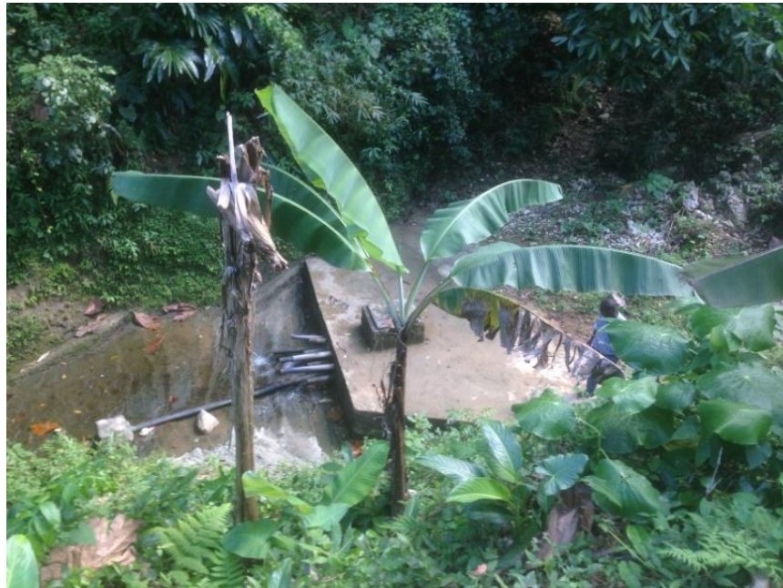
Captage source Guichard
