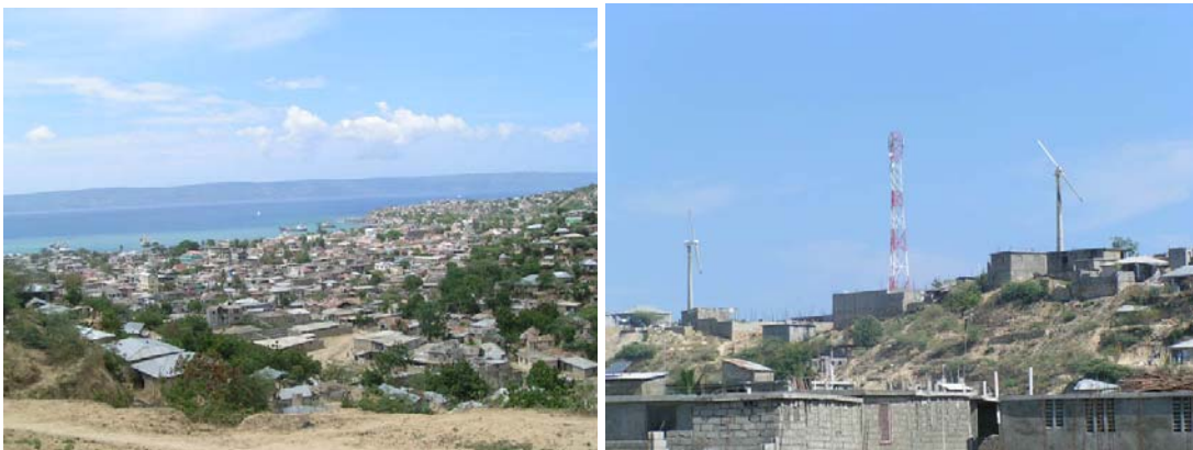
Figure A3. Port-de-Paix and its nonoperational wind plant
